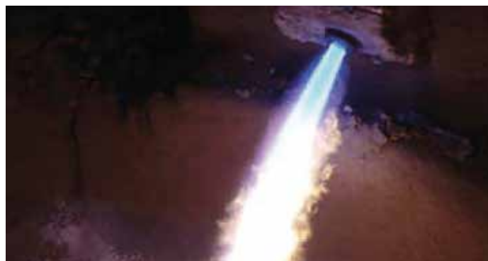
Blue colored flame due to the poor mixing of oxygen and natural gas.
